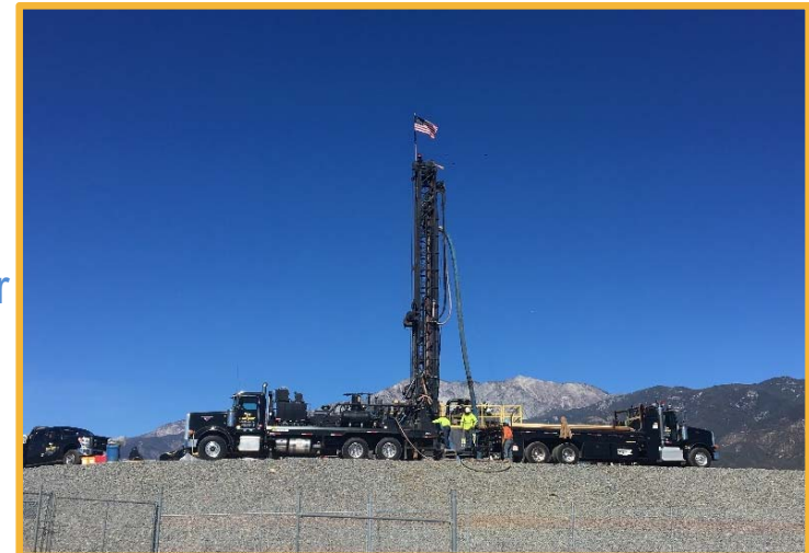
Monitoring Well Construction
