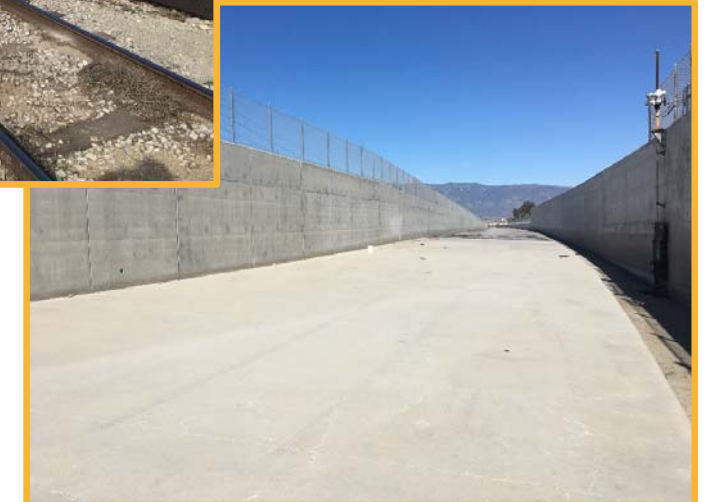
San Sevaine Channel near Jurupa Basin
