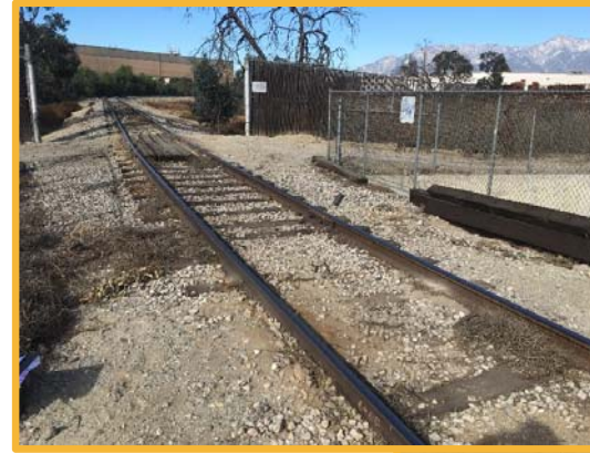
Rail Road Spur - Pipeline
