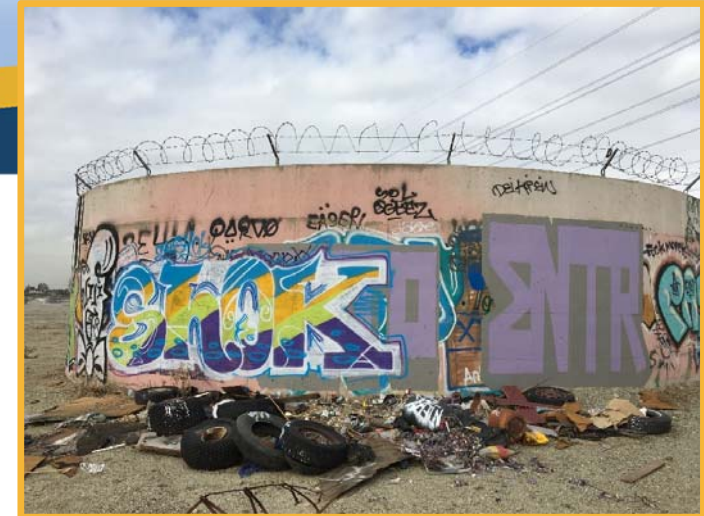
Abandon Treatment Tank
