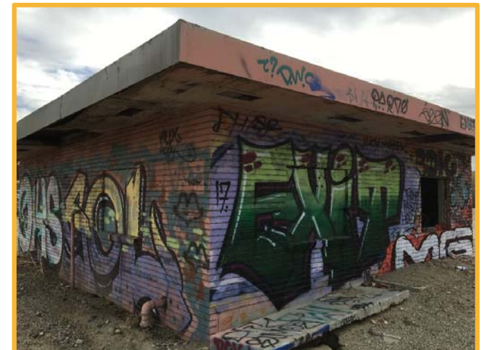
Abandon Pump Building
