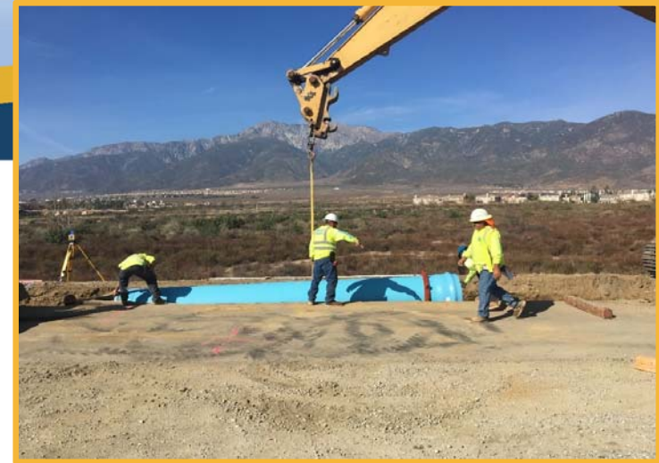
30-Inch PVC Install
